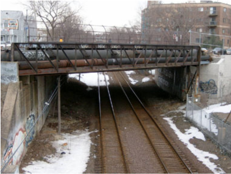
Looking at Webster Street bridge with existing train tracks below
