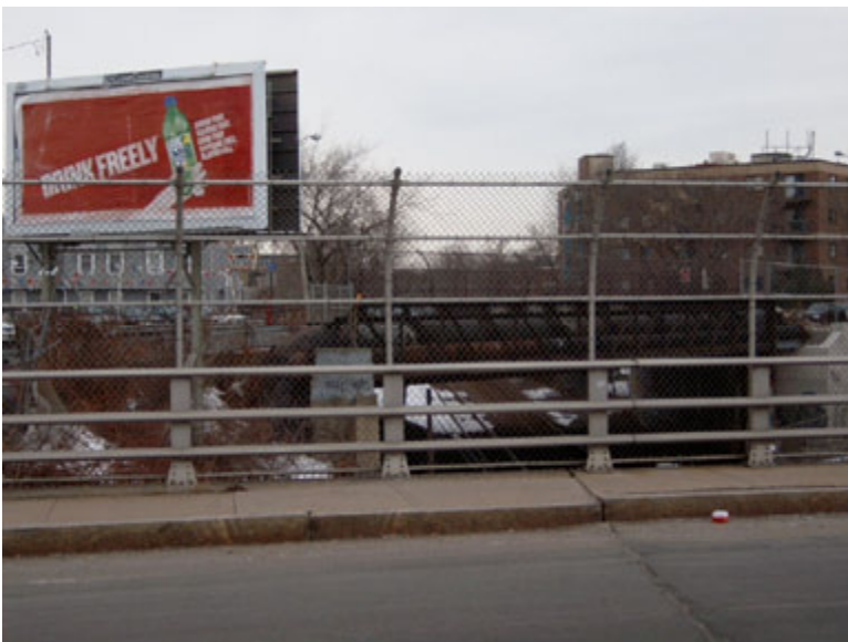
Looking from Prospect Street Bridge over project site to Webster Street bridge with train tracks below
