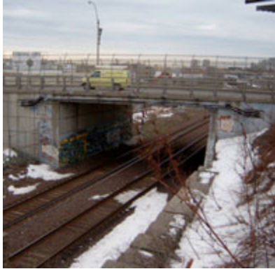
Looking east: Prospect Street crossing over existing train line
